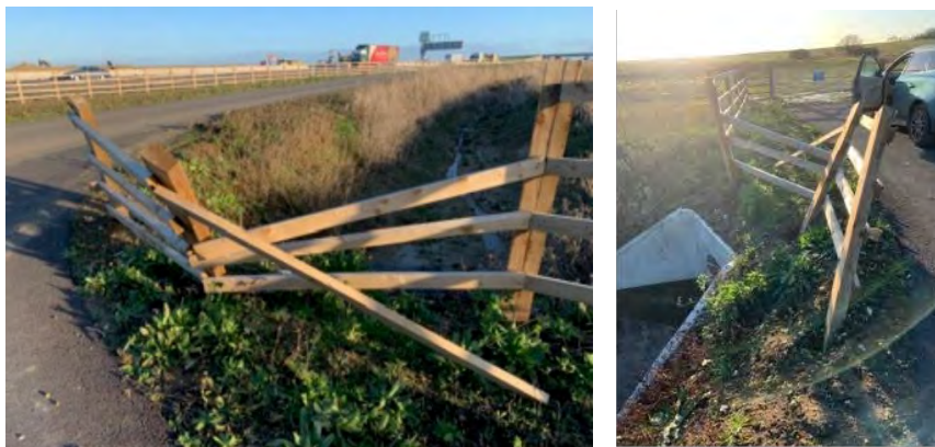
Figure 2 – A14 accommodation works
