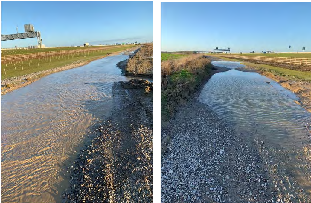
Figure 9 – drainage issues along the A14
