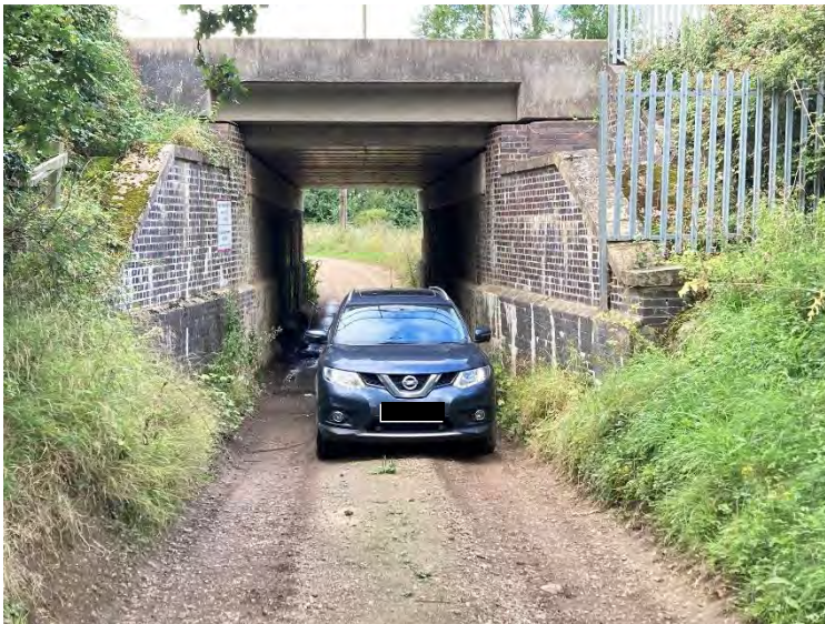
Figure 5 – East Coast Mainline underpass
